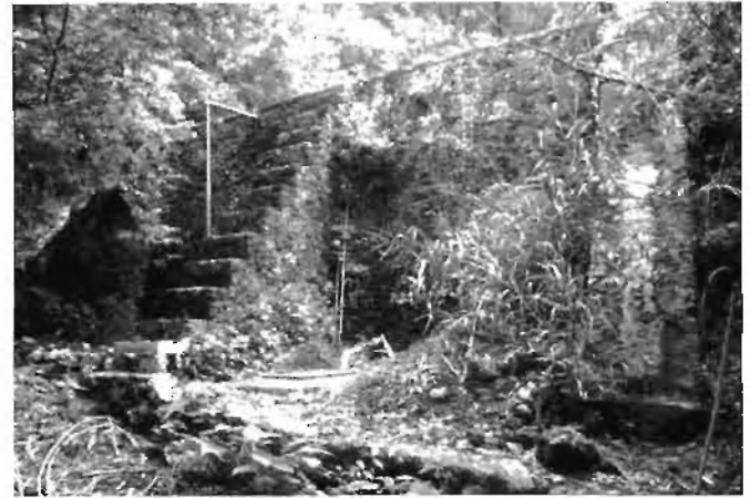
The "presa piramida" (pyramid dam)—a 100,000 gal (380 m 3 ) cistern made by sealing off the space between two walls of bedrock with stone and cement. This construction is difficult to seal perfectly leak-tight, which is important if you don't have water to add to the cistern for eight months.
