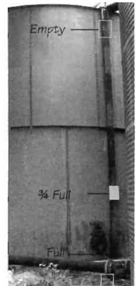
Bought float-type level indicator.
