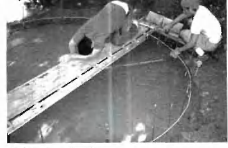
6. Leveling the floor to 2% slope and finishing.
