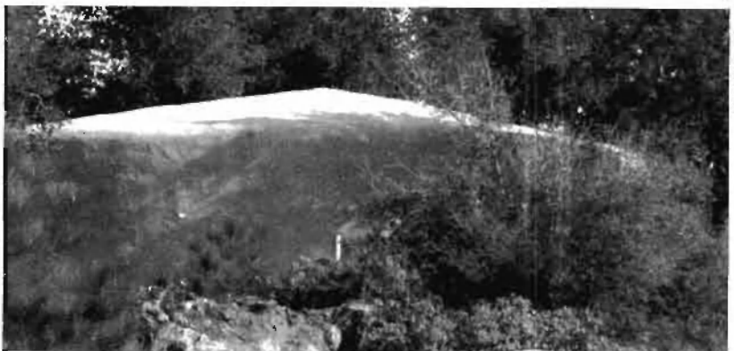
A completed 40,000 gal (150 m 3 ) tank.
