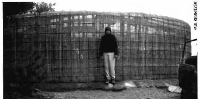
40,000 gal (150 m 3 ) ferrocement tank, ready for plaster.
