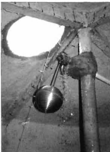
Float valves automatically shut off the water when the tank fills.
