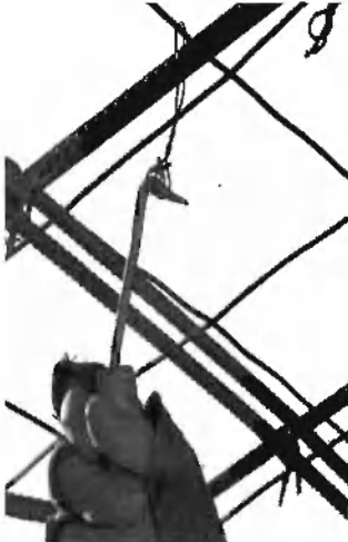
Tying off welded wire mesh.
