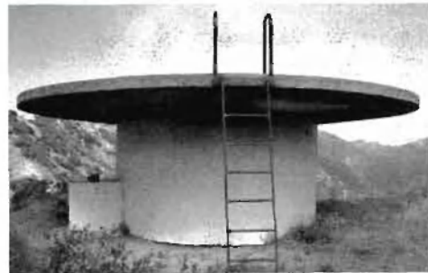
A 1,000 gal (3.8 m 3 ) pre-cast concrete septic tank.
