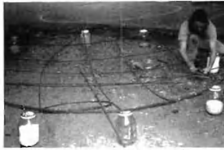
10. Bending and tying off the roof rebar.
