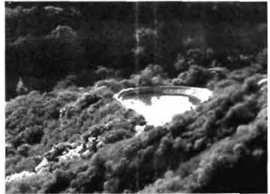
A concrete-lined storage pond excavated into the spine of a ridge above an avocado orchard. It is filled by water pumped up from a creek diversion through a few hundred feet of 4" pipe.
