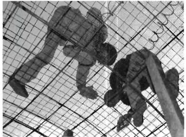
Tying off expanding metal lath on roof with pneumatic hog ring pliers.
