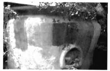
21. Check out your plaster colors carefully, with big swatches... we measured to the gram on a postal scale, then multiplied for big batches.
