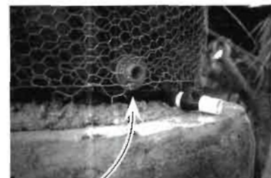
250 gal (1 m 3 ) HDPE drinking water tank with new bulkhead fitting outlet and chicken wire ready for stucco. (See also Plastic Tank Drain Retrofit, p. 60.)
