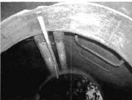
Ladder made of 1/2", epoxy-coated, grade-60 rebar integrated in a ferrocement water tank. This choice of rebar reduces the two main problems with rebar ladders: bent steps (grade 60 is half again as strong as standard grade-40 rebar) and rusting away, which can render the ladder unsafe as well as impact the structural integrity of the tank wall.
