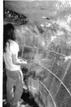
11. Tying off lath (inside) and chicken wire (outside); first make a hook on the end of the wire, push it through...
