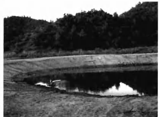
Construction of a 100' (30 m) diameter embankment pond in the Cuyama Valley, California. It is filled by gravity with water from a creek diversion, through a mile of 2" pipe. It is used for swimming and emergency storage.
