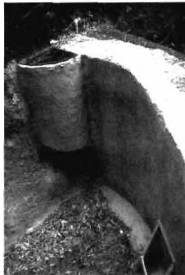
A 12,000 gal (44 m 3 ) mortar and rock diversion at the base of a waterfall in Mexico.
