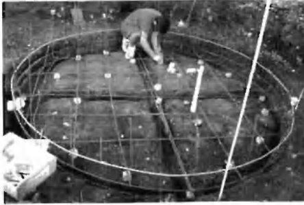
4. Concrete filling "X" of trenches makes grade beams to reinforce floor.
