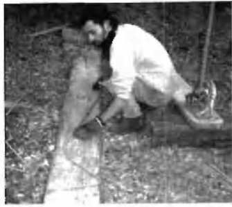
7. Bending the rebar verticals.
