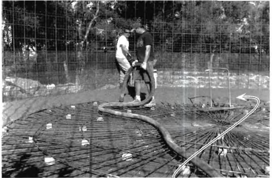
Pumping and spreading concrete for the floor.
