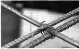
Double rebar tied.
