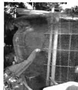
12. Then pull the hooked end back through, grab it with linesman's pliers, twist, then cut the tie off your spool of wire.
