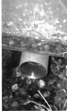
Welded drain from the outside, ready for plug and concrete work.
