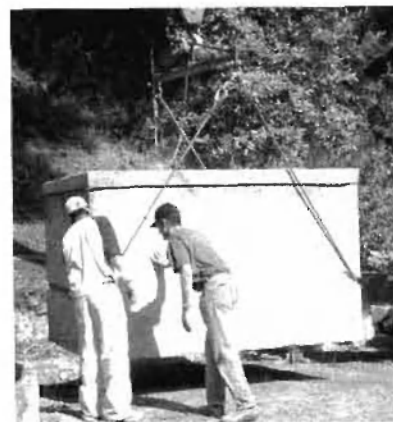
A 1,000 gal (3.8 m 3 ) pre-cast concrete septic tank.
