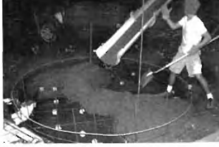
5. Pouring the floor.
