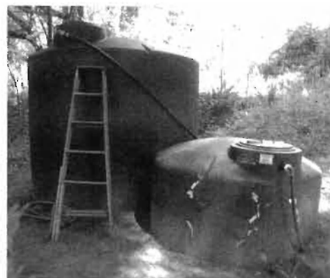
Different height HDPE water tanks. Shorter tank is for drinking water; taller tank is for all other uses. The systems aren't connected at all.
