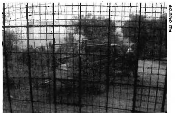
Close-up of wall armature; 1/2" rebar on 1' centers, two layers of 6" x 6" mesh, offset to make 3" squares, sandwiched between expanded metal lath on one side and chicken wire on the other
