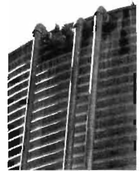
Separate inlets from two wells, and an overflow all the way at the top of a riveted, corrugated galvanized tank.
