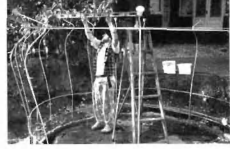
9. Placing the first rings and then verticals.
