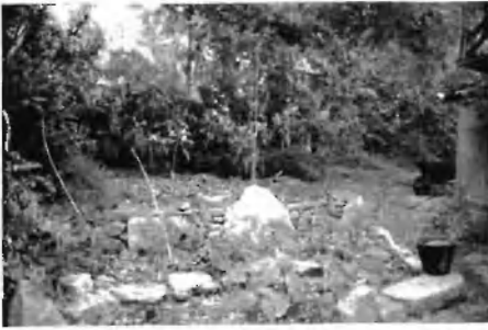
1. The site, before digging.
