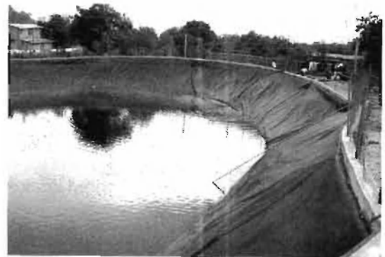
Runoff-harvesting storage pond for a village in Mexico. This EPDM-lined pond is filled through a mile (1.5 km) of 2.5" HDPE line from a seasonal creek. It fills for about four months and is used primarily for laundry during the long dry season.
